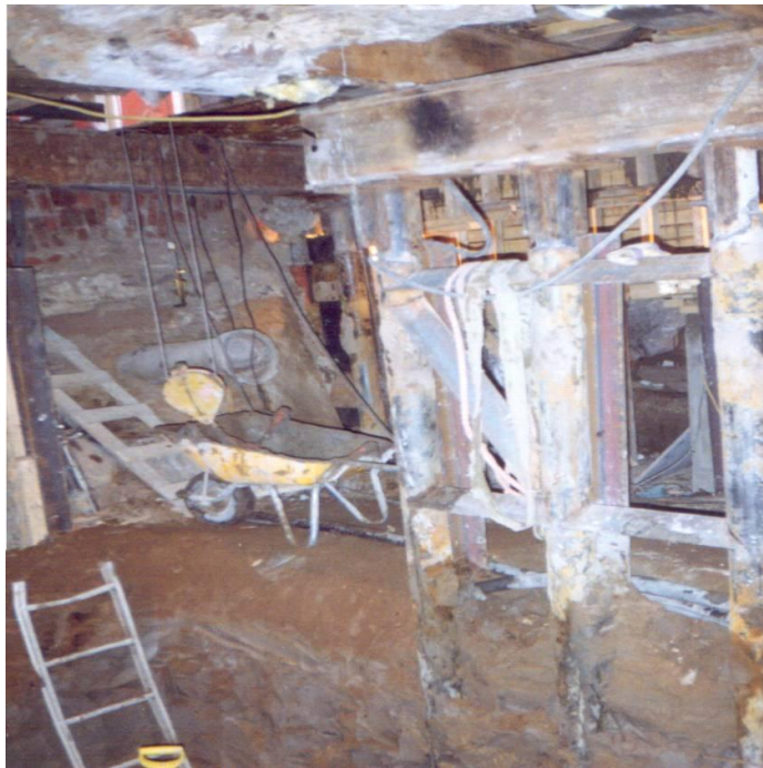
Picture 6. Digging work under old structures of Aleksanterinkatu 4 - 10.
