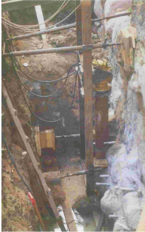
Figure 5. Simple screw driving equipment for drilled spiral piles.
