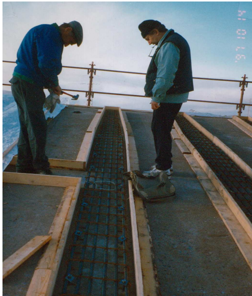
Photograph 3. Formwork and reinforcement of upper parts of beams. Mr. Kokko of the contractor firm Kokkoma Ltd and the writer.
