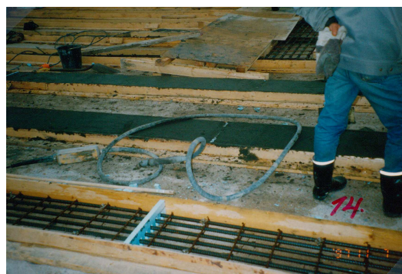
Photograph 4. Concrete pouring of the upper parts of the beams.
