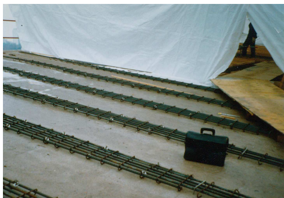
Photograph 2. Reinforcement ready for the upper parts of the beams and part of winter hall.
