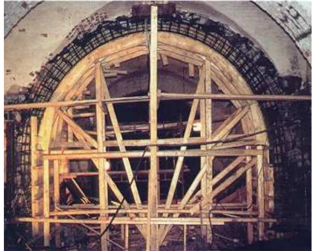
Figure 6: South wall. Rock and earth anchors. Photograph 4: Reinforcement of concrete arch.
