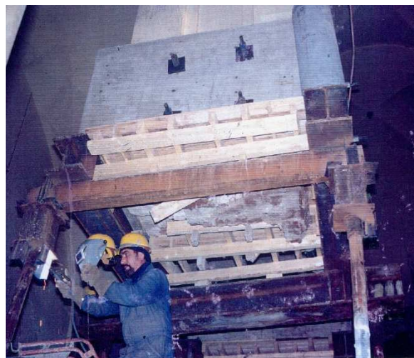
Photograph 3: Eastern stair column. Old brick column. Pretensioned concrete plates. Temporary steel supports.
