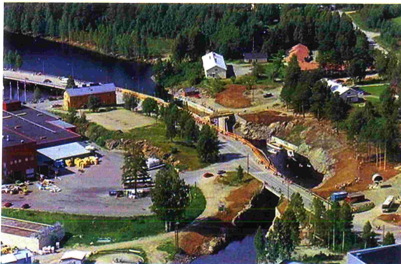
Fig.: 2: Juankoski: built lock and part of the channel
